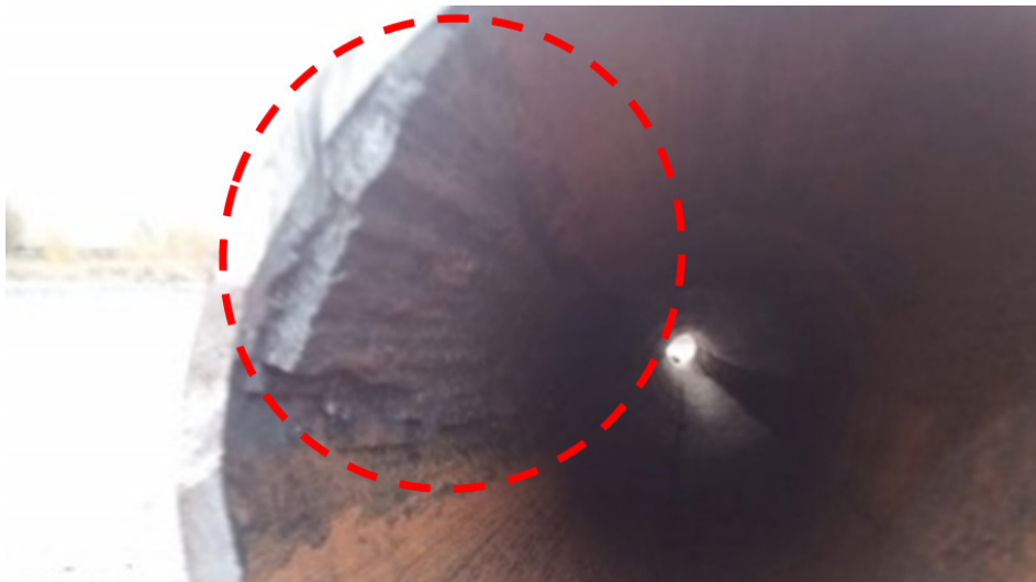
Figure 2. Internal Fouling
